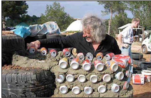
Figure 3: Michael Reynolds building a structure with cans bottles . Source: Bernard , 2008
