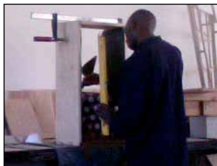
Figure 33: Building the bottles wall. Source: Personal collection
