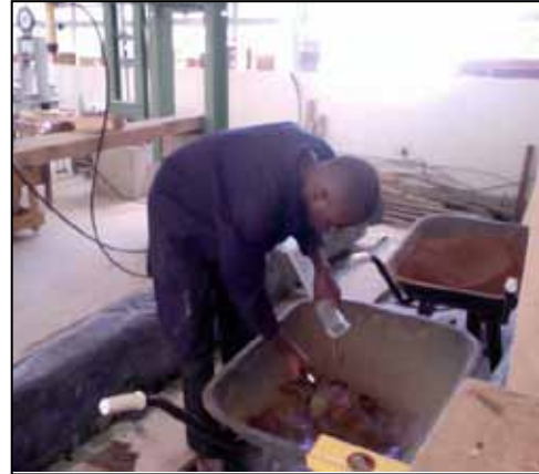
Figure 32: Mixing the mortar
